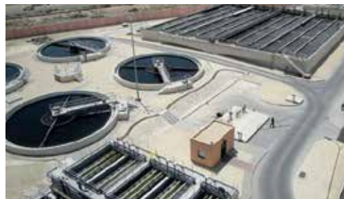
Sewage Treatment Plant Supply of Tiles Guocera, Refin
