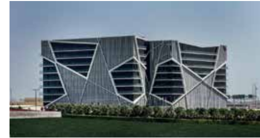
Al Baraka Bank - Bahrain Bay Supply of Sanitary ware Duravit, Hansgrohe, Sonia
