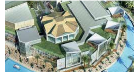
Mall of Delmunia Supply of Sanitary ware & Mixer Duravit, Hansgrohe, Conti+, Italia Granite, Niro Granite
