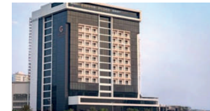
The Grove Hotel - Amwaj Supply of Tiles, Sanitary ware Duravit, Tece, Axor, Porcelanosa
