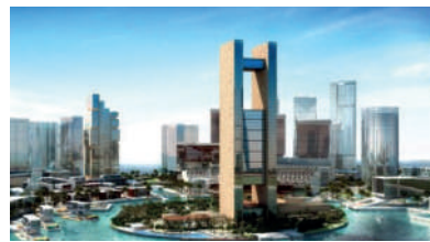
Four Seasons Hotel - Bahrain Bay Supply of Sanitary ware Duravit, Geberit
