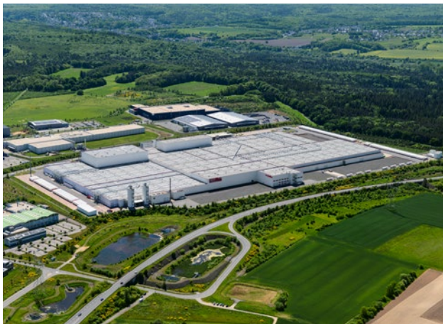
Plant V in Saarlouis
